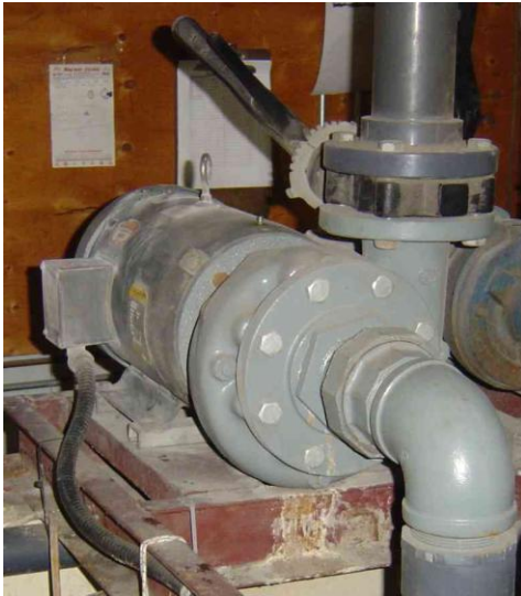
Figure 4: Centrifugal Pump
