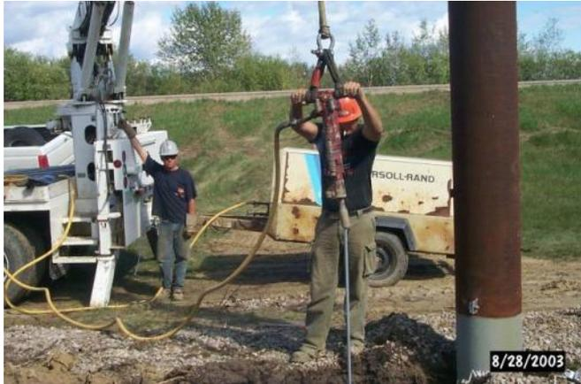
Installing ground rods
