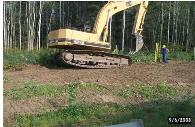
Tension (proof) testing anchors
