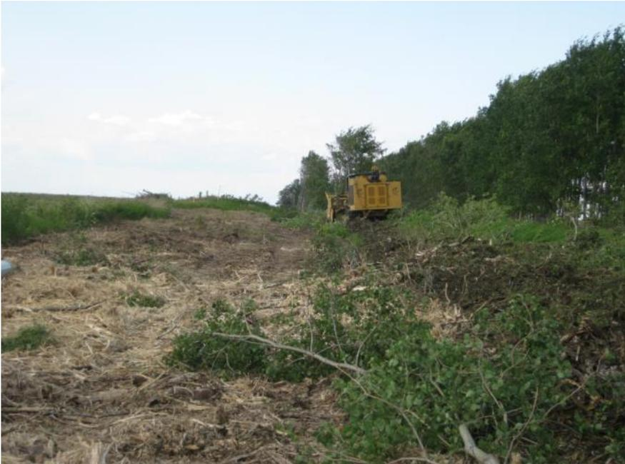
Drum mulcher clearing right-of-way
